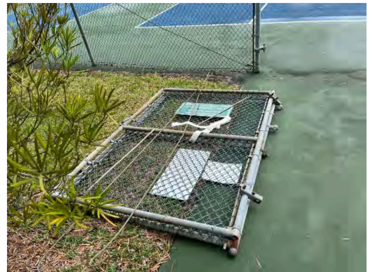
The old fence around the court is removed.
